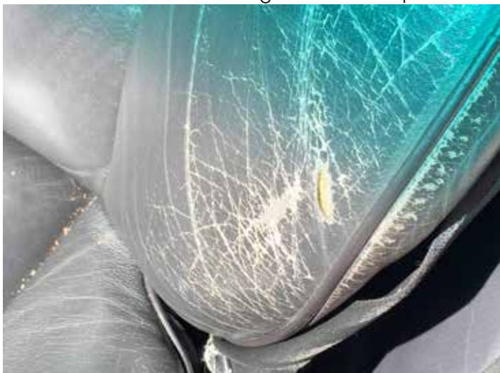
Cracks left unchecked will develop into holes. All photographs by the author.
