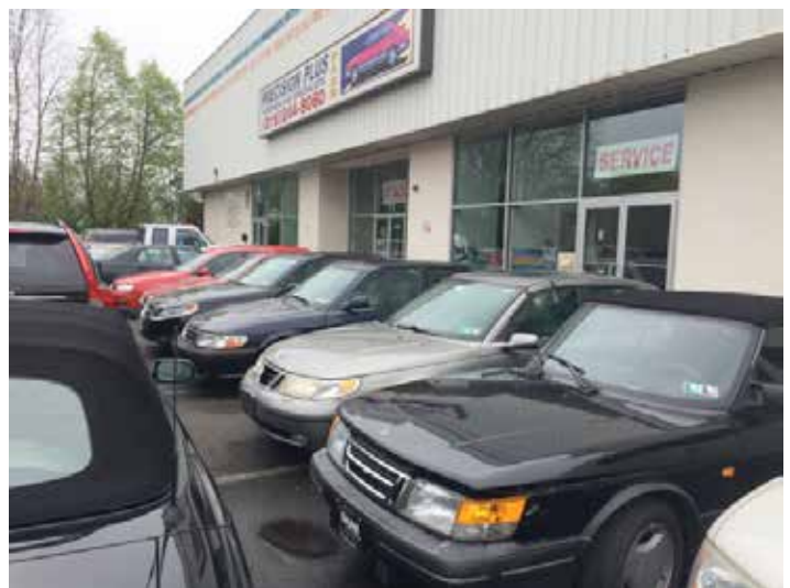
The Precision Plus building in Trevose, PA Photographs provided by the author.
